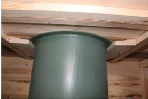
The height of the waste chute can be adjusted by sliding up or down. If the chute is too long, the excess part can be cut off with a saw.
